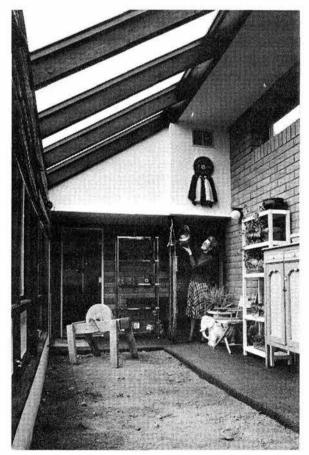
GREENHOUSE INTERIOR with planting area. Note slump rock trombe wall at right.
